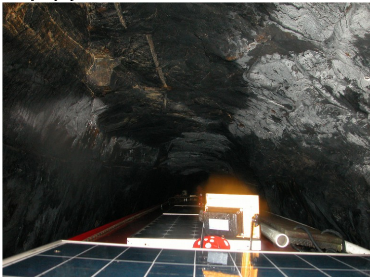
Shot-holes in the Millstone Grit roof. Photo: Jenny Drake
