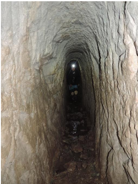
Left: Much of the adit was cut as a superb coffin level.
