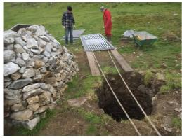
Grille being manipulated into place. Note pile of waste rock
