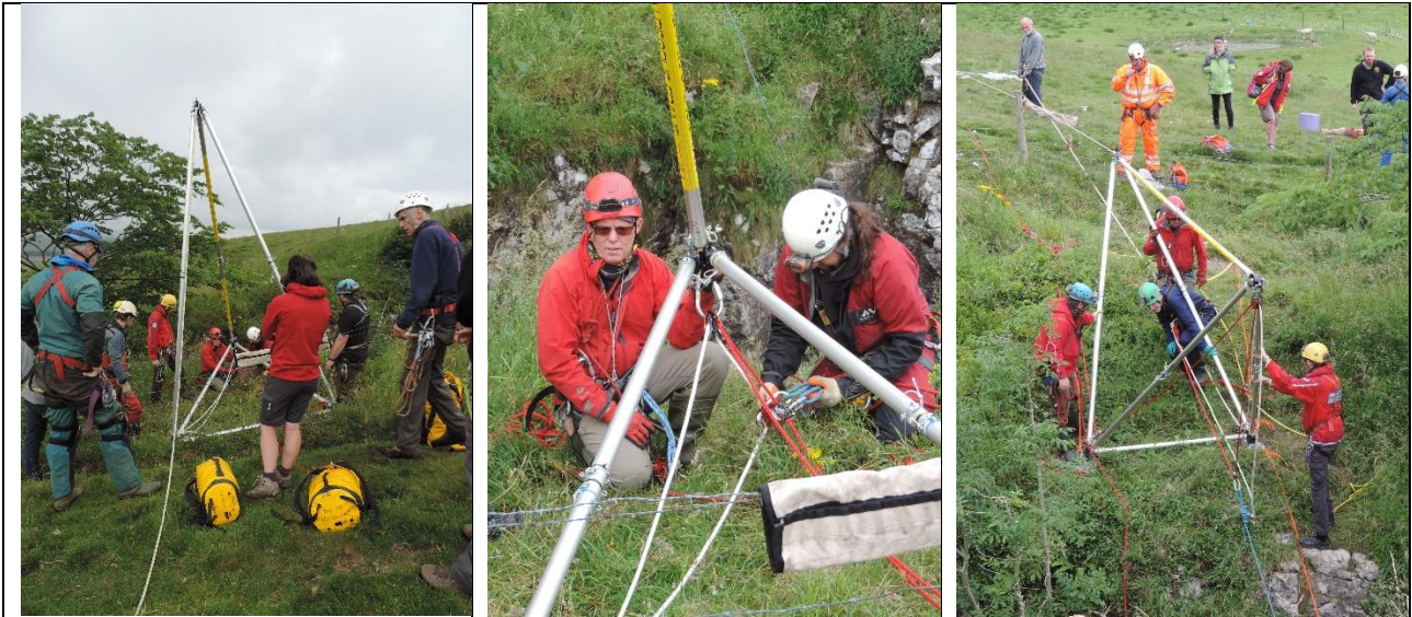
Assembling the Larkin Frame close to the shaft edge, before moving it into position, and securing with ground anchors and ropes. Everyone near the shaft was securely belayed, and everything was under the watchful eye of the Safety Officer. All photos: Steve Knox
