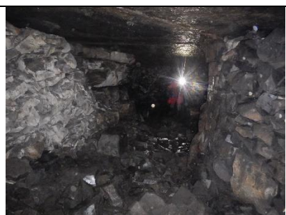
A typical stretch of passage with pack-walls 'supporting' the roof.
