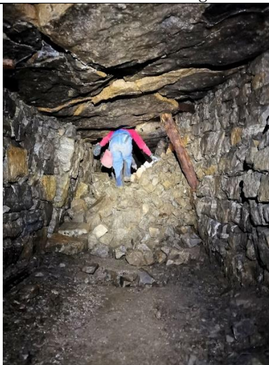
Collapsed pack-walls, due to the pressure of the rock above, almost blocked some routes.
